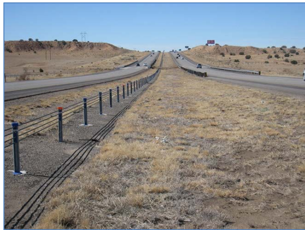
Image 1. Incident site looking south; note gentle down-slope to north end of bridge. (NIOSH photograph)
