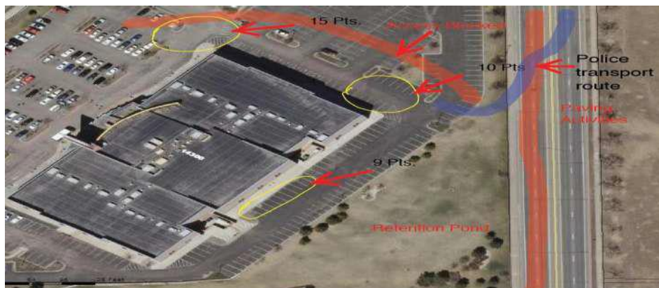
Figure 11. Police Car Access and Egress 17
